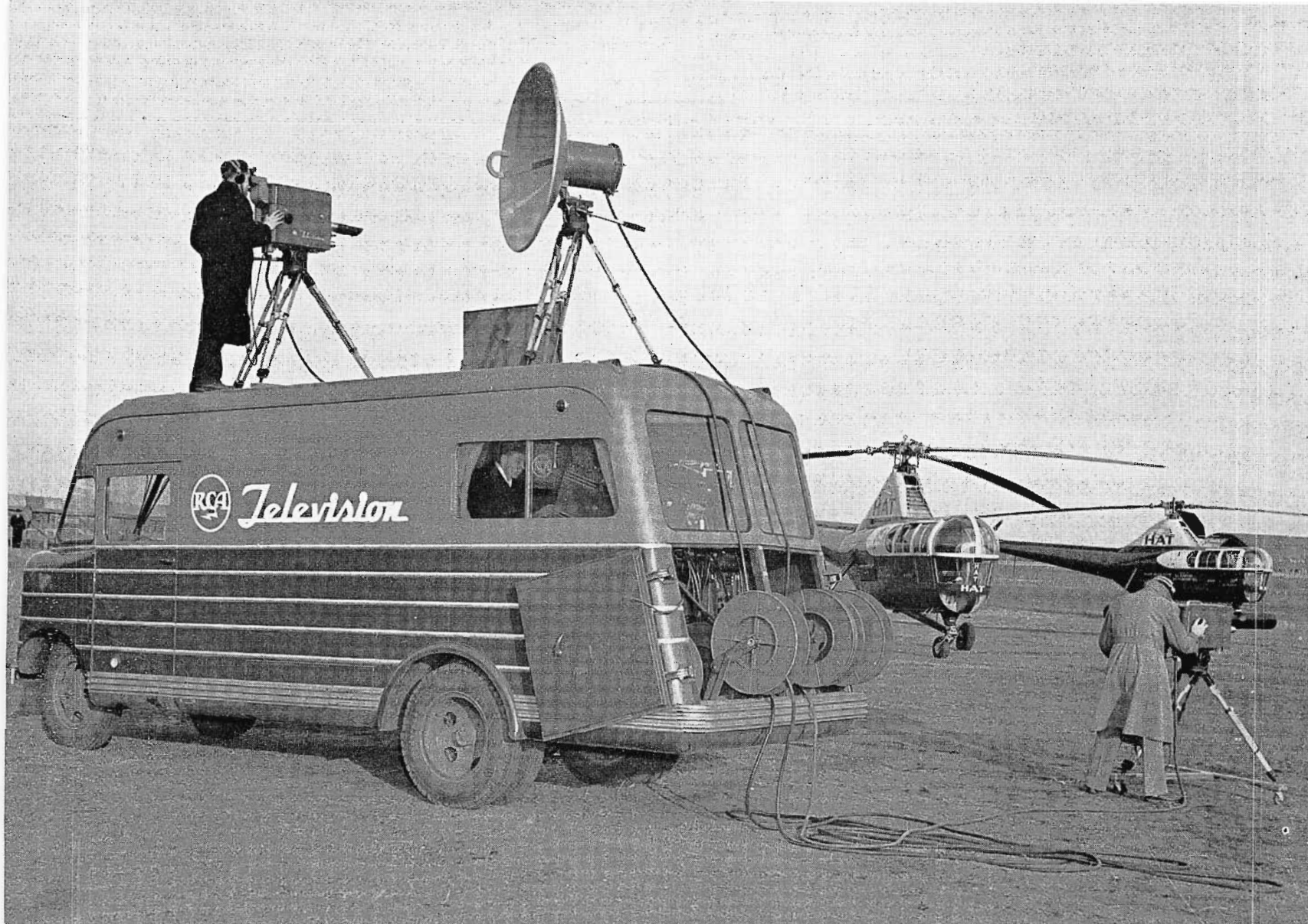
FIG. 1. The TJ-50A Mobile Unit (shown here at Camden Airport) provides both transportation and control space for standard field equipment. Cameras may be operated from the roof of the unit or placed as much as 1000 feet away.
