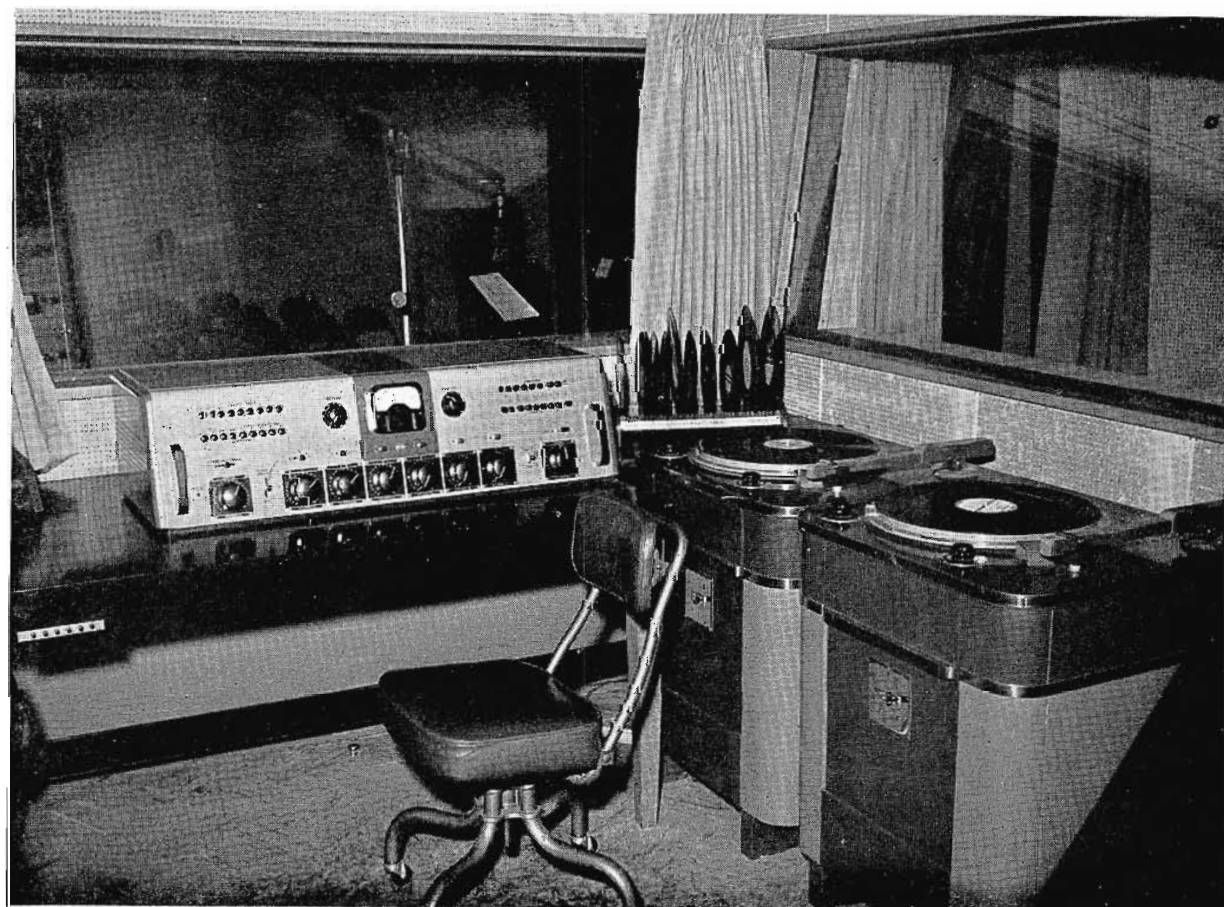
FIG. 4. WMIN's Control Room showing their RCA 76-B2 Console and 70-C2 Turntables.
