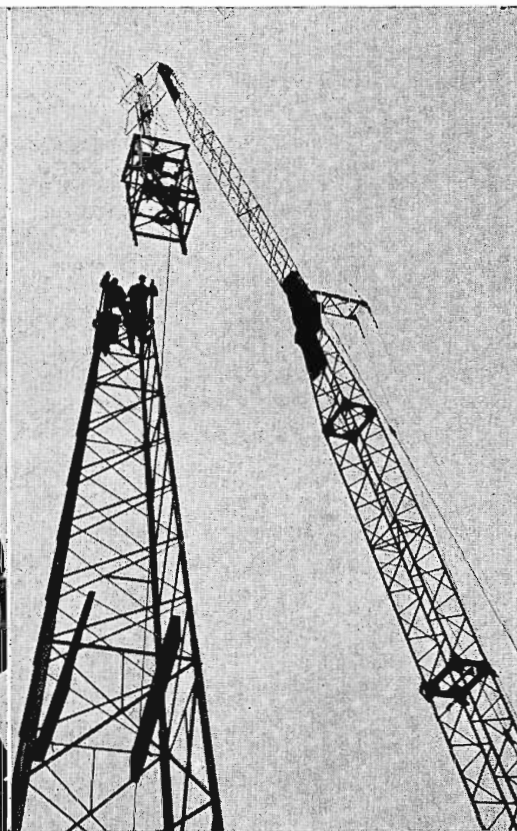
FIG. 6. This shows the turnstile and top section of the 100-foot tower being lifted into place.
