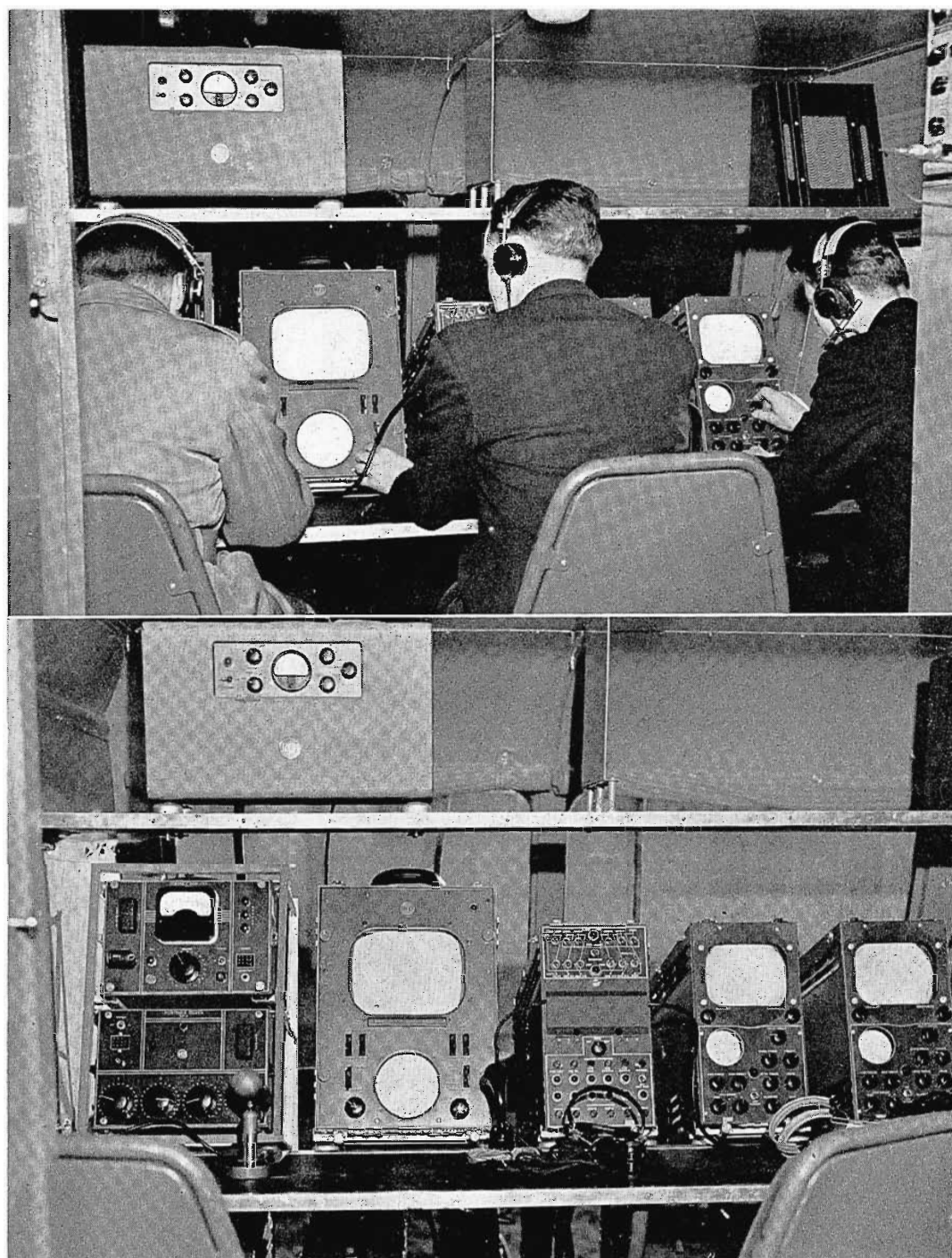
FIG. 5. (right, above) Operating position has seats for audio operator, director and video operator.
